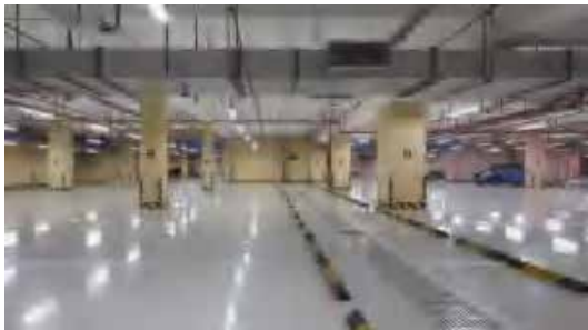
Underground car parks
